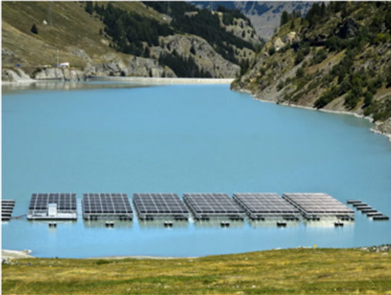
Solar panels float on a mountain lake in Switzerland. The first such system was installed in 2008. Gunter Fischer / Education Images / Universal Images Group via Getty Images
