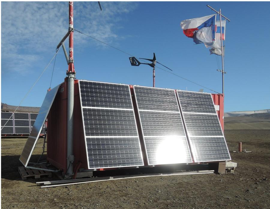
Fig. 5. PV modules installed on the container.
